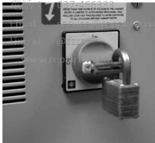
Fig 1.6 Disconnect Handle Positions – Shown OFF, With Padlock
