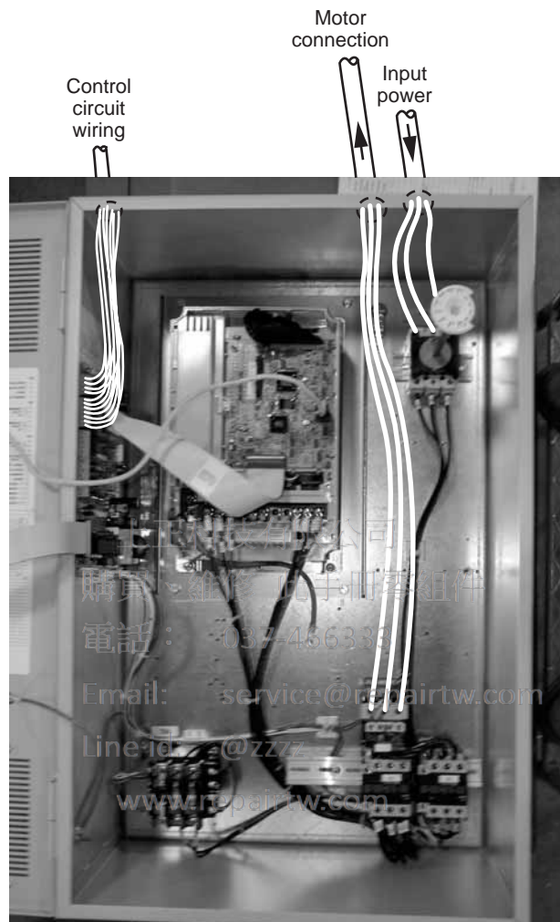
Fig 2.5 Typical Wall Mount Enclosure
